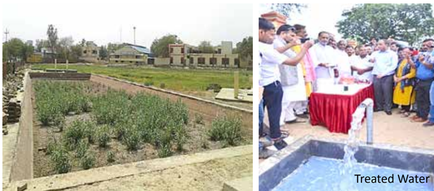
Out-scaled ICAR-IARI wastewater treatment facility at Pandit Deen Dayal Upadhyay Village, Farah (Mathura)
